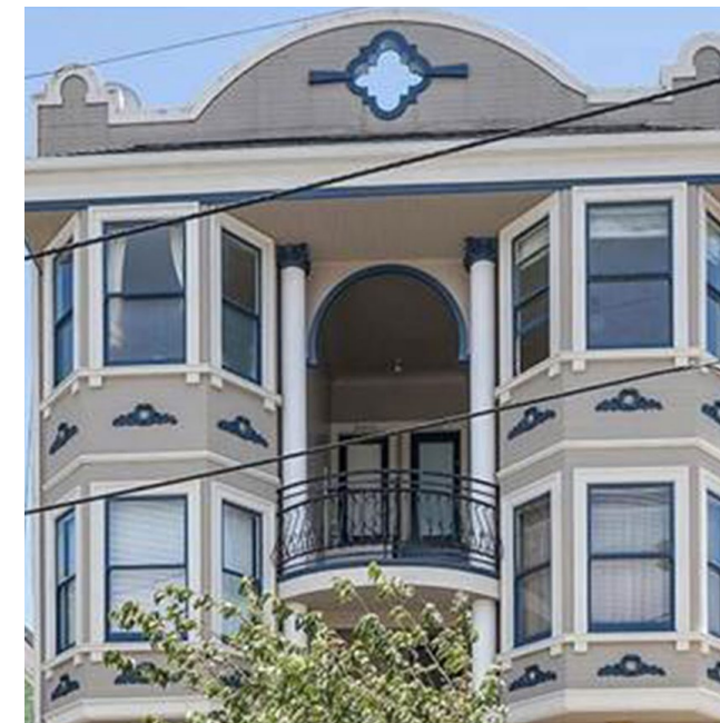
A San Francisco apartment building that received energy and comfort upgrades through the BAMBE program.
