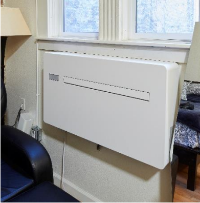
Left: A package-terminal heat pump (PTHP). Right: Central condensing water heaters.
