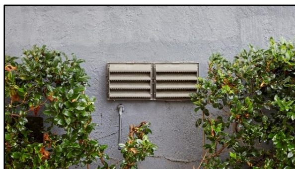
Above: An Innova package-terminal heat pump (PTHP)
