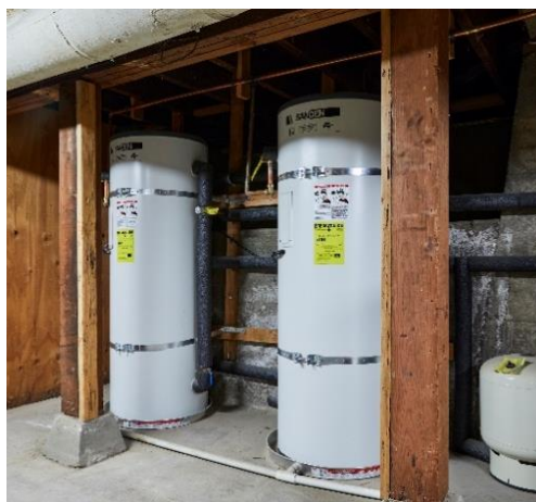
A central heat pump water heater with 2 tanks provides reliable hot water to the entire building.
