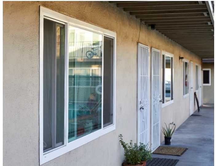
New dual-pane windows were installed throughout the property
