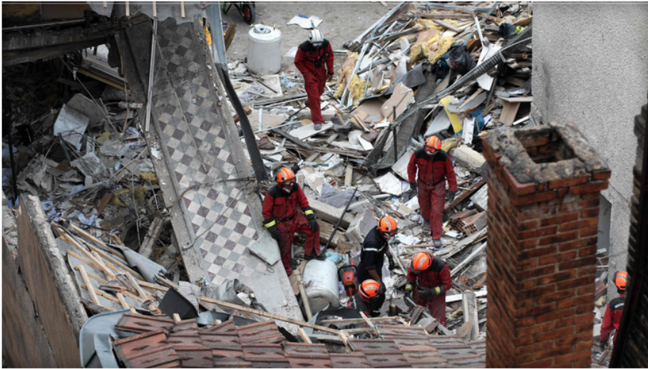
French firefighters work in the rubble on Pierre Palliot Street in Dijon, France, after a gas explosion destroyed a building on Sept. 16, 2016. / ROMAIN LAFABREGUE/AFP/GETTY IMAGES
